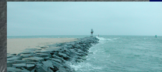
North Jetty (looking east) traps sand that would otherwise feed AI beaches
