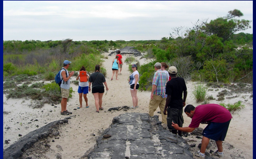
Remnants of Baltimore Boulevard, the intended main drag of the ill-fated "OB" development (2012)
