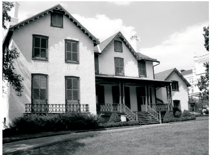
Front entrance to the cottage
